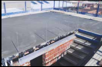
Double clay brick & concrete upper floor (not prefabricated pod)
